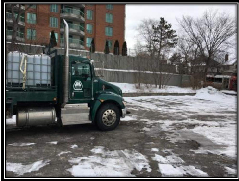
Photograph 3: View of drilling activities at MW17-01, facing southwest (Feb 11, 2017)
