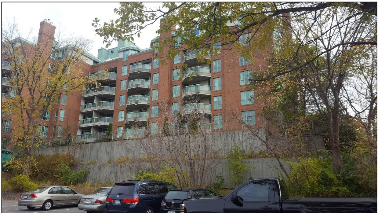
Photograph 8: View of adjacent property to the east, view northeast (October 27, 2016)
