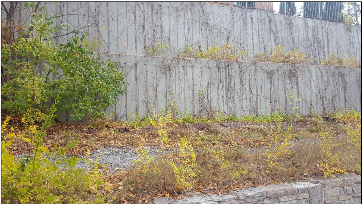
Photograph 10: View of retaining wall at east property boundary (October 27, 2016)
