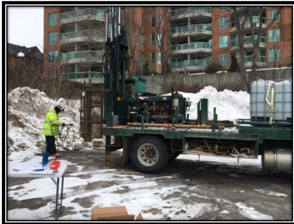
Photograph 2: View of drilling activities at MW17-01, facing northeast (Feb 11, 2017)
