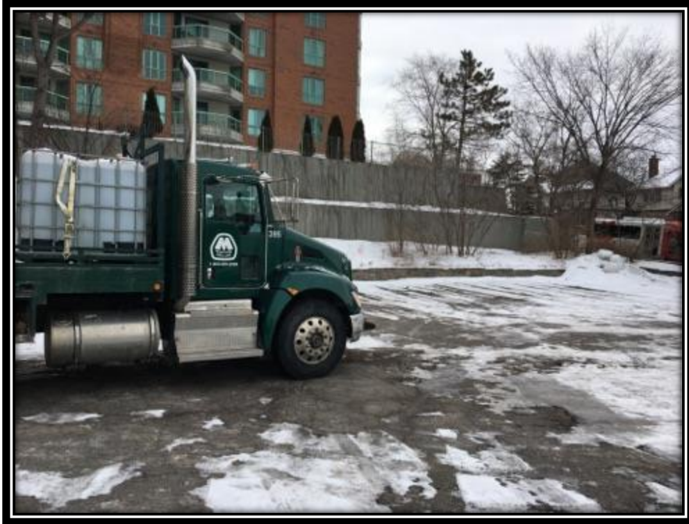
Photograph 3: View of drilling activities at MW17-01, facing southwest (Feb 11, 2017)
