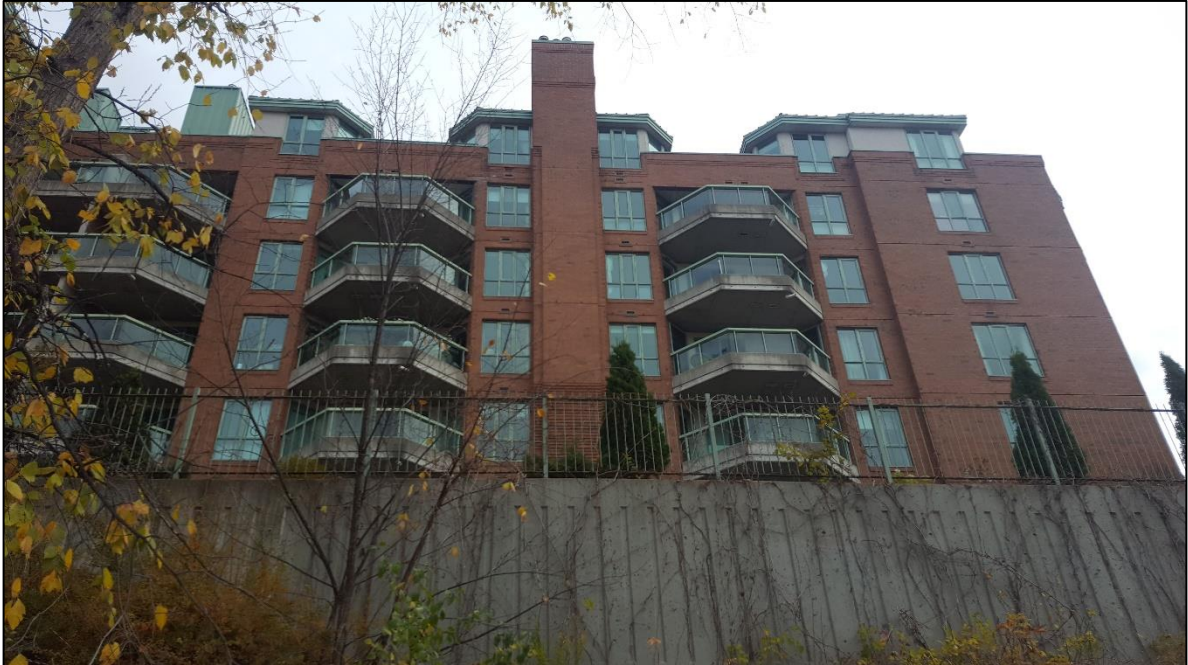
Photograph 9: Adjacent property to the east of Site (October 27, 2016)
