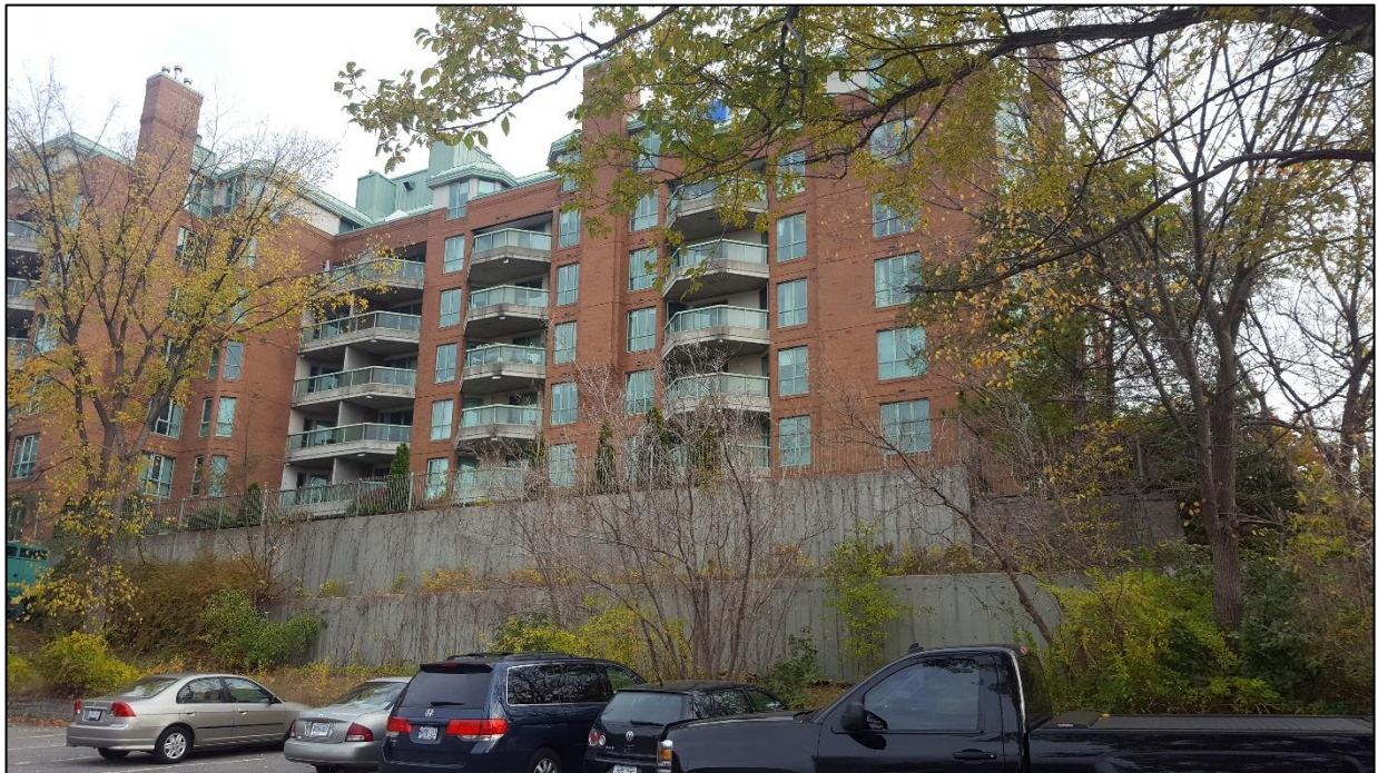
Photograph 8: View of adjacent property to the east, view northeast (October 27, 2016)
