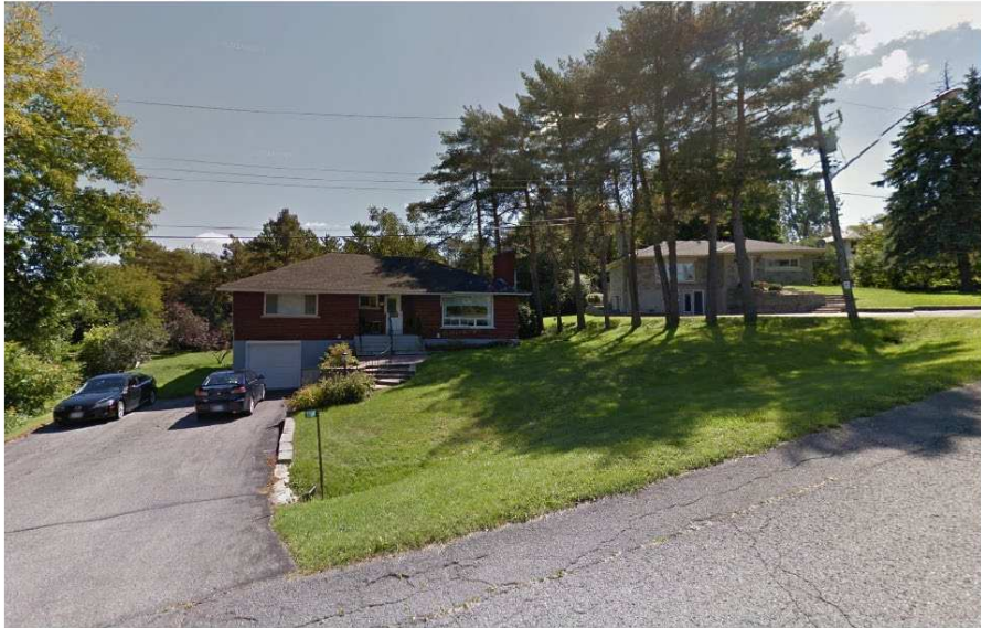
Facing 1164-1166 Highcroft Drive
