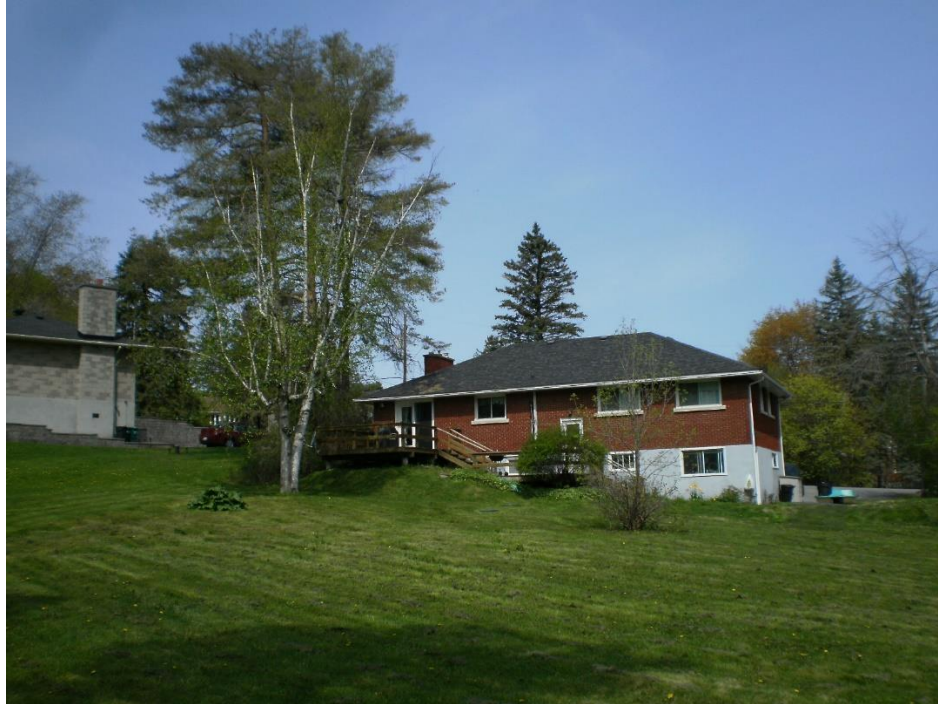
Photo 5 – South portion of 1164 Highcroft Drive. From southeast corner of the site view looking north to residence to be removed
