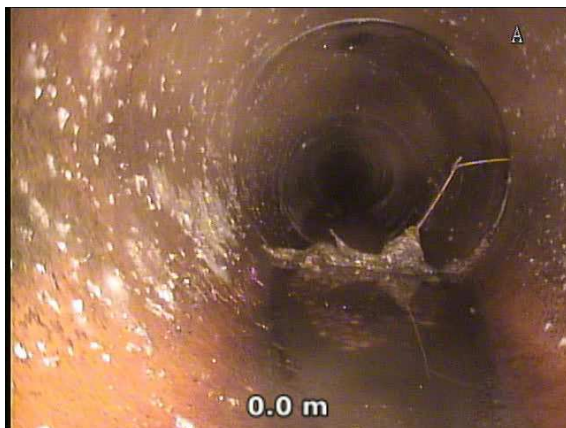
Figure 6 – 375mm diameter vitrified clay tile sanitary sewer between MHSA1 and MHSA2
