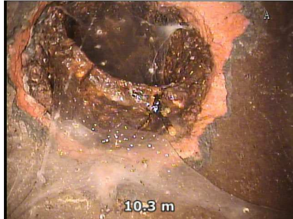
Figure 9 – 100mm diameter pipe connection at 11 o'clock (10.3m from MHS A1)
