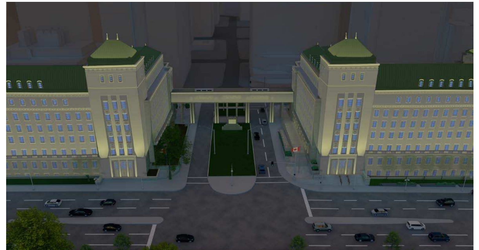
Ensemble Night Lighting
