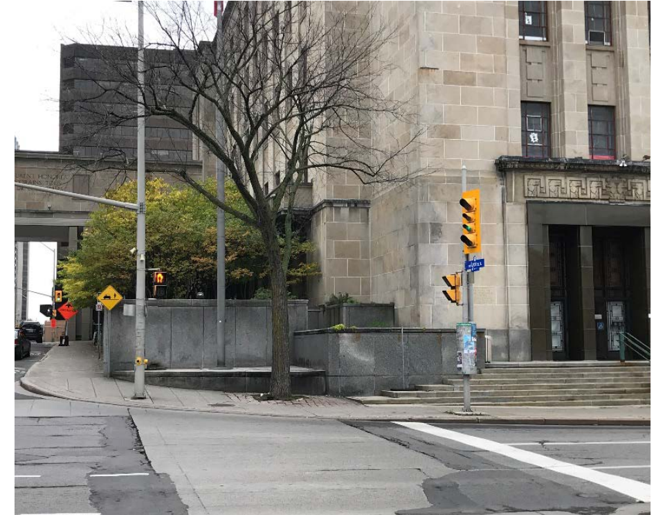
Interlocking Terraces at North-East Corner
