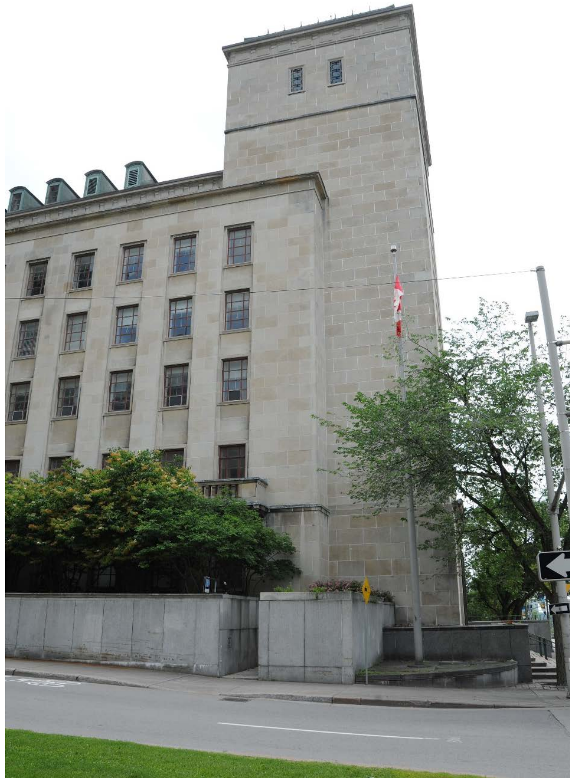
East Facade - Existing Condition
