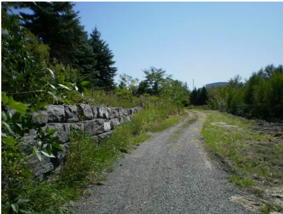
Photo 8 – Access trail, retaining, wall, berm and coniferous plantings on and adjacent to the east edge of the site. View looking south from the north property line
