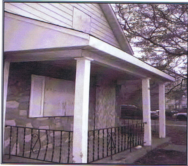
Photo 3 – Site Building C (west elevation).
