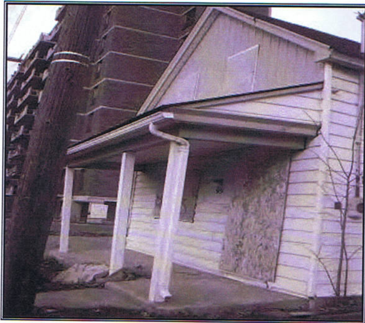
Photo 1 – Site Building A (west elevation).
