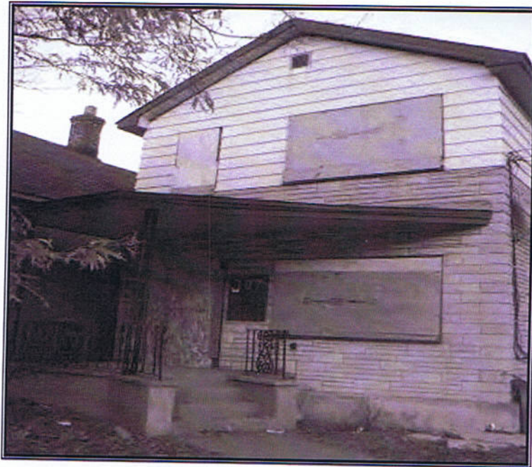
Photo 4 – Site Building D (west elevation).
