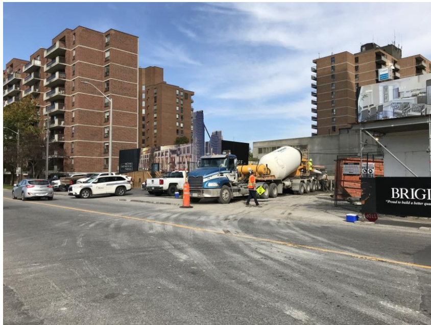
Photo 1: Overview of the Site from Parkdale Avenue, facing northeast.
