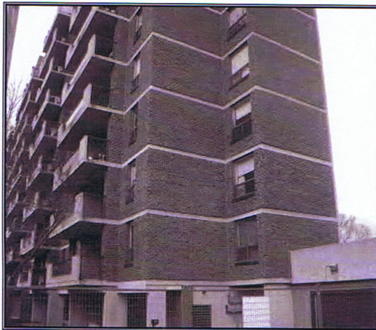
Photo 6 – Adjacent property located north of the Site.
