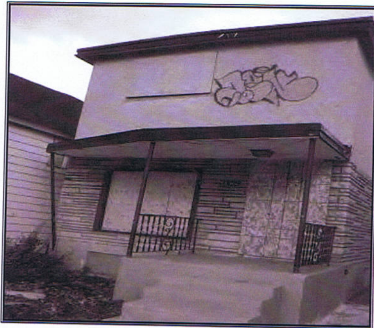
Photo 2 – Site Building B (west elevation).
