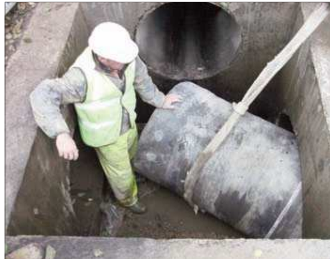
24" CheckMate® is easily installed in a municipal sewer.
