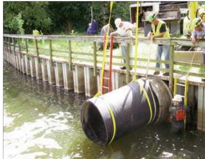
48" CheckMate® installed in a storm sewer drain to stop backflow from flooding a residential area.
