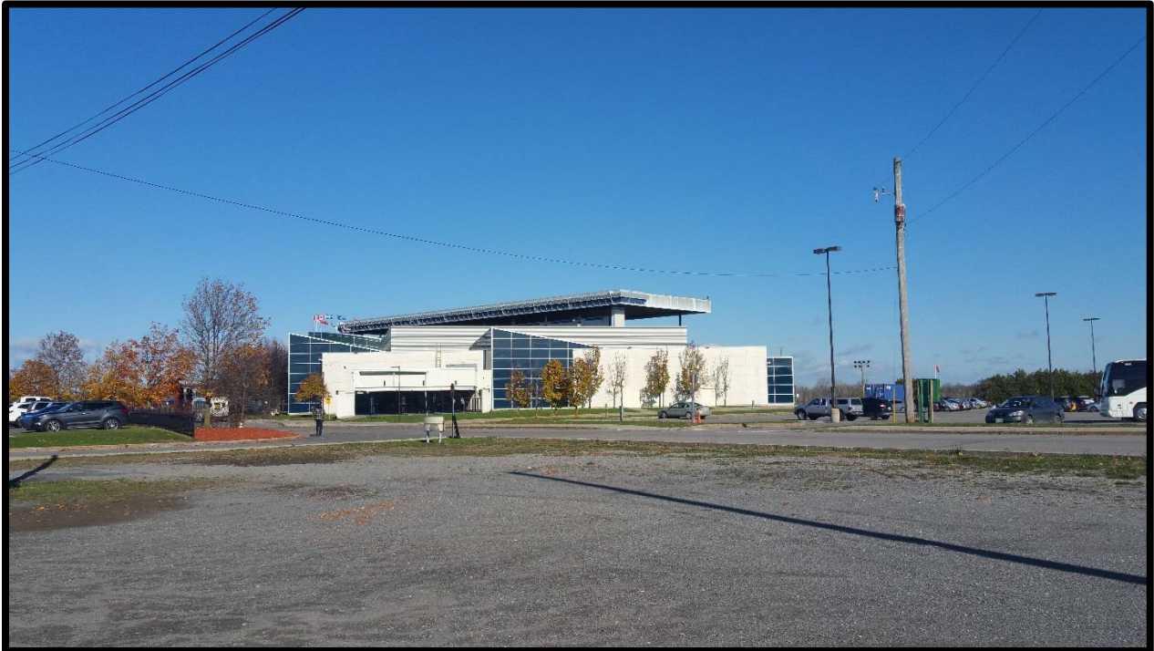
Photograph 1: View of the southern portion of the site, facing northeast. Photograph illustrates a gravel parking lot in the area of the residential dwelling and the Rideau Carleton Raceway building.
