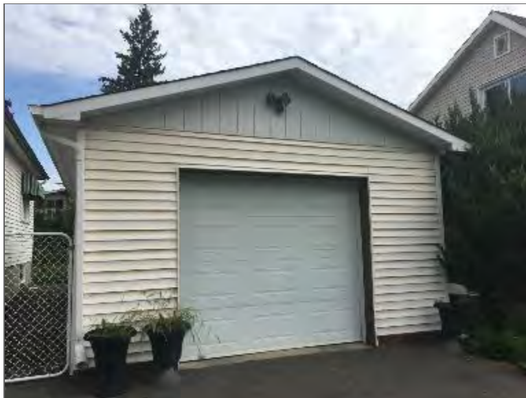
Photo 4 – Detached garage building associated with Site Building A.
