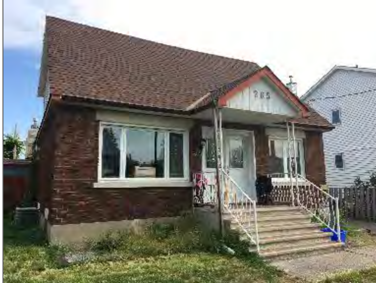
Photo 5 – Site Building B (south elevation).
