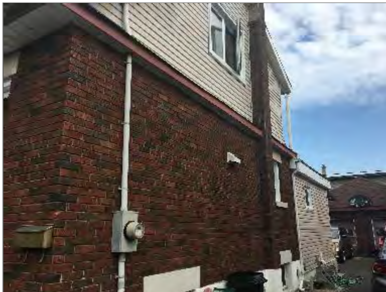
Photo 6 – Site Building B (east elevation).
