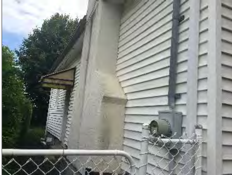
Photo 3 – Site Building A (west elevation).
