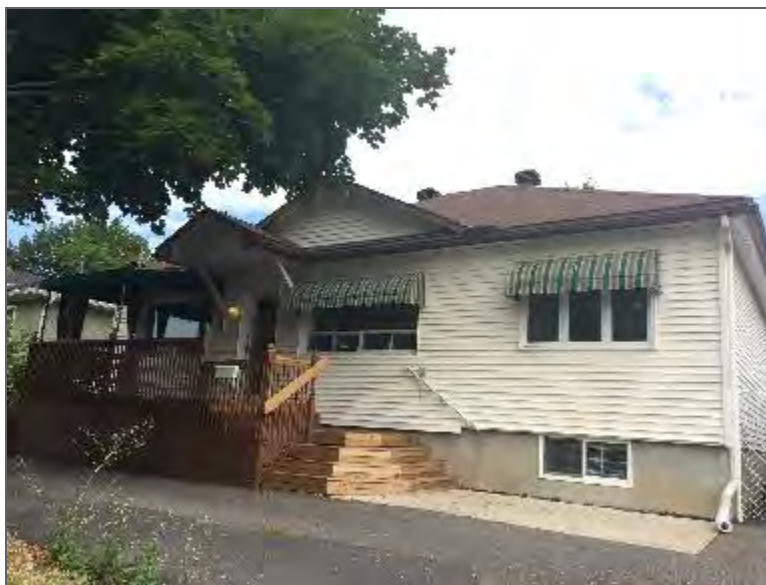
Photo 2 – Site Building A (south elevation).
