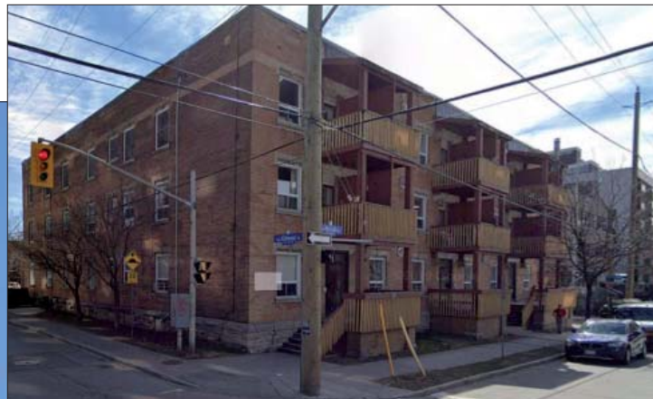
(Figure 5) Gainsborough Apartement Building
