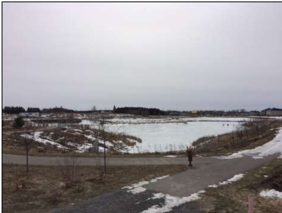
Photograph 6: View of the northwest corner of 5505 Fernbank Road, looking southwest from the south end of Tapadero Avenue. The Storm Water Management Pond associated with the Monahan Drain can be seen in the center of the photograph.
