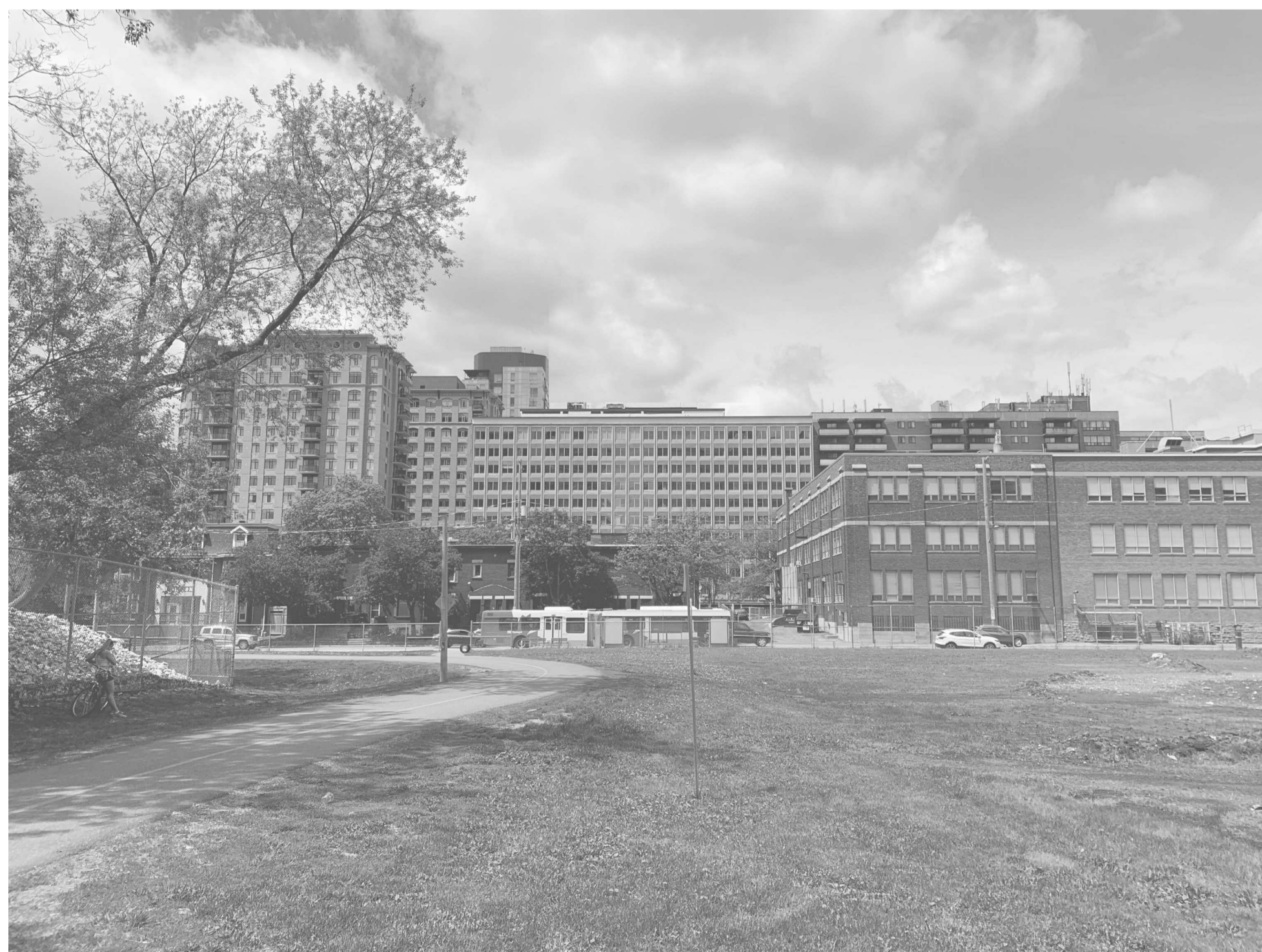
EXISTING VIEW FROM SOUTH
