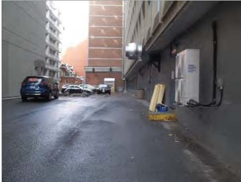
Photo 5 – Site Building (northwest elevation).
