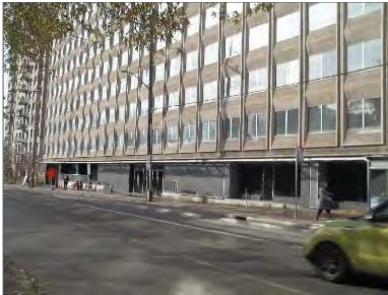
Photo 4 – Site Building (southeast elevation).
