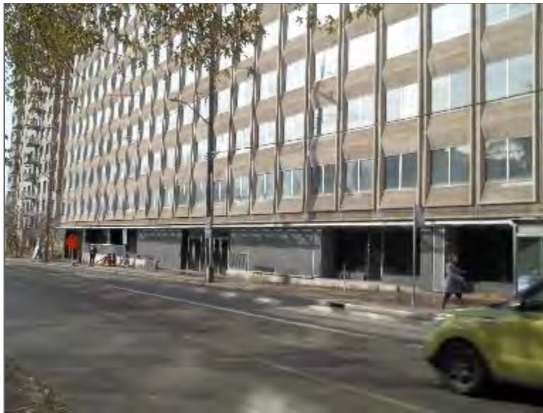
Photo 4 – Site Building (southeast elevation).
