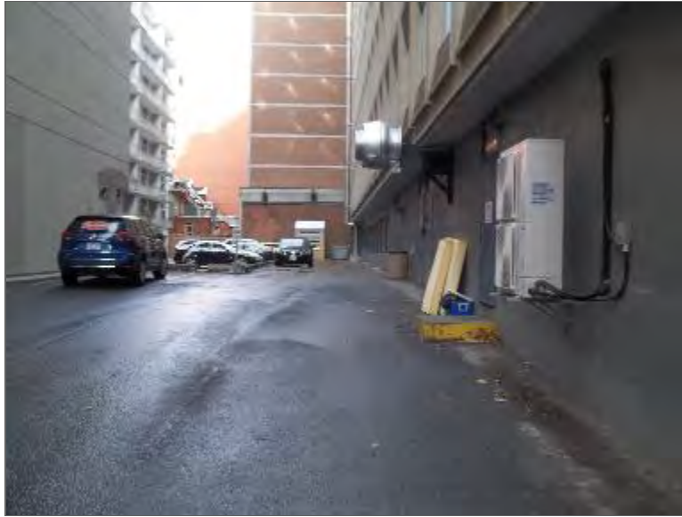
Photo 5 – Site Building (northwest elevation).
