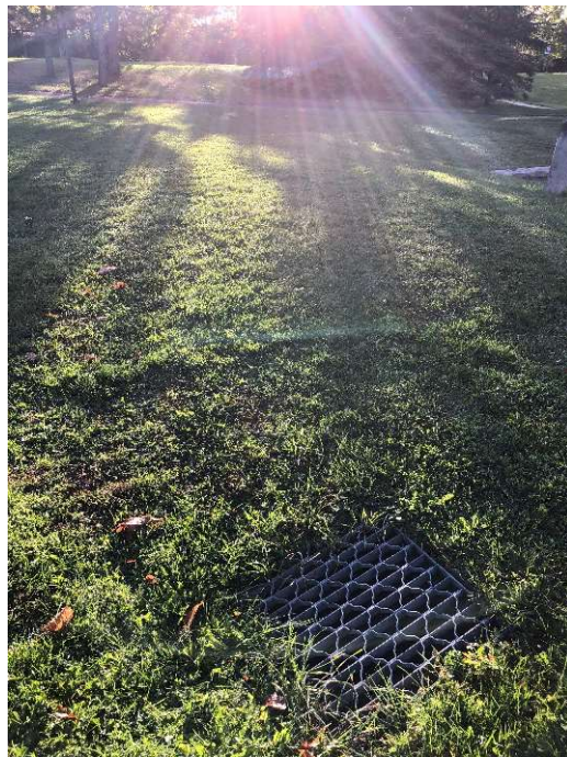
6. View of stormwater grate, located near the centre of the Phase One Property
