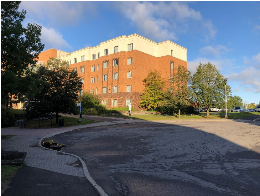
4. View of adjacent residence to the west (Leeds House)
