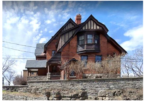
Figure 8: 593 Laurier Avenue, corner (south and east) façades of existing building. (Google)
