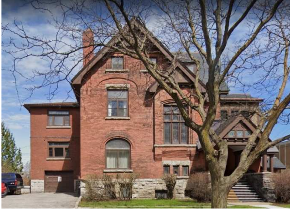
Figure 7: 593 Laurier Avenue, front (south) façade of existing building. (Google)
