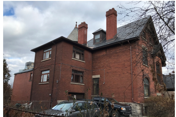
Figure 10: 593 Laurier Avenue, front and side (south and west) façades of existing building. (RMA)
