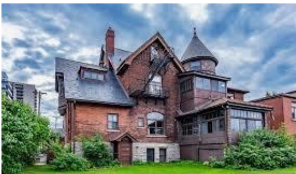
Figure 11: 593 Laurier Avenue, rear (north) façade of existing building. ( https://bennettpros.com/ )
