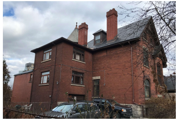
Figure 10: 593 Laurier Avenue, front and side (south and west) façades of existing building. (RMA)
