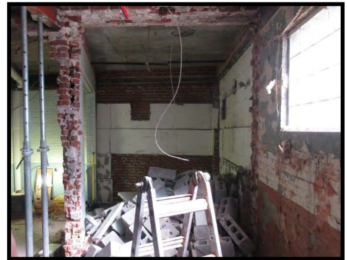
Right: Former upper floor building entrance at the southeast end of the CBN building.
