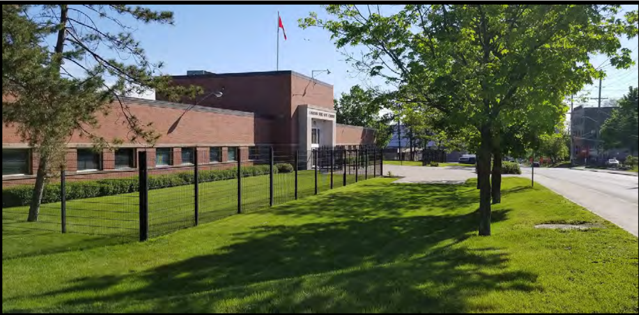
Looking northeast at the southern portion of the Phase One Property, as seen from southwestern corner of the Phase One Property.
