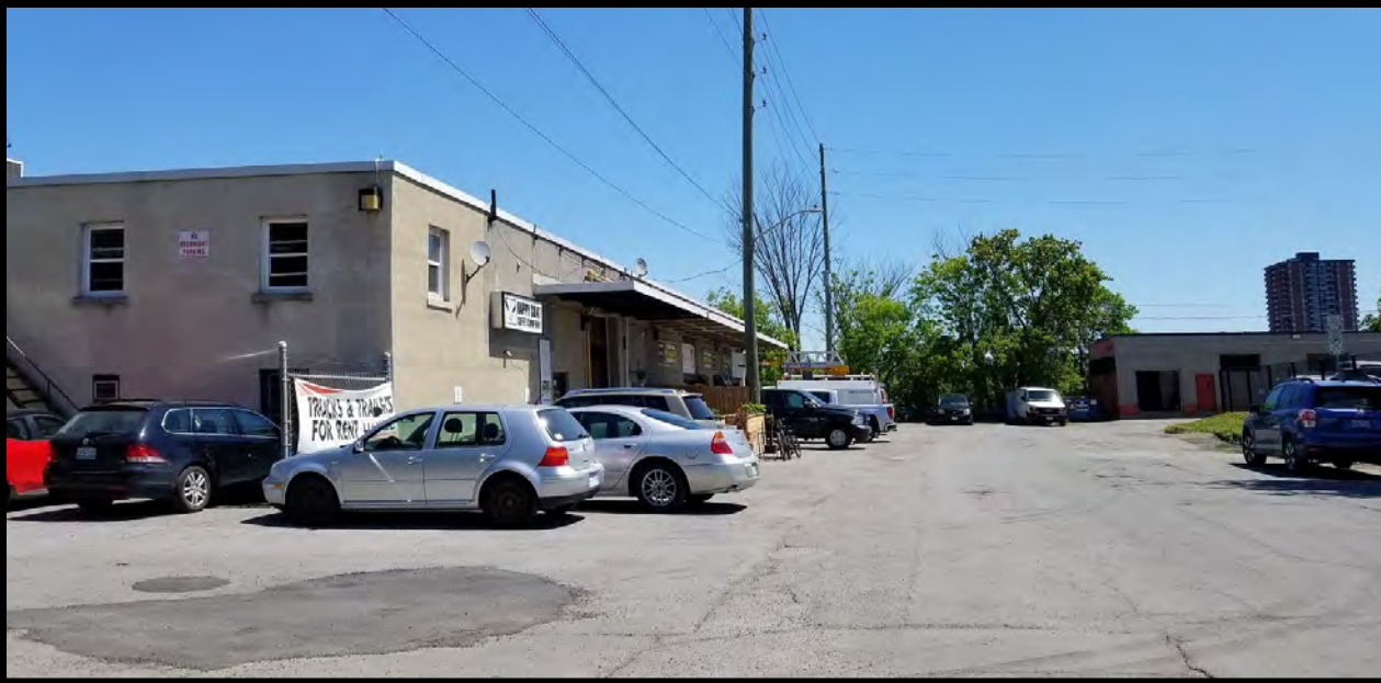
Looking northeast at the northeastern portion of the Phase One Study Area, as seen from Laurel Street near the middle of the Phase One Property's northern boundary.
