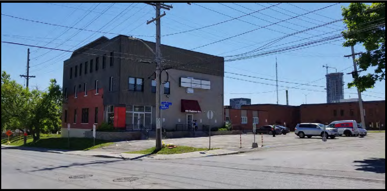
Looking southeast at the southeastern portion of the Phase One Study Area, as seen from just outside the southeastern corner of the Phase One Property.
