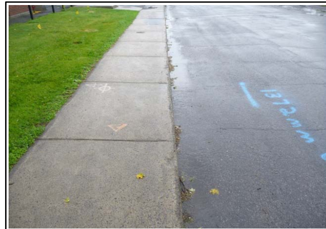
Photo 2 - 1372mm Water Main Adjacent to Sidewalk
