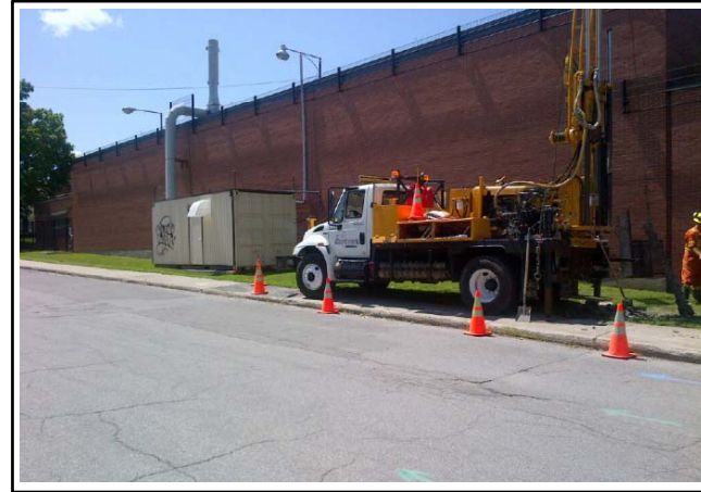
Photo 6 - Drill Rig Setup at MW5
