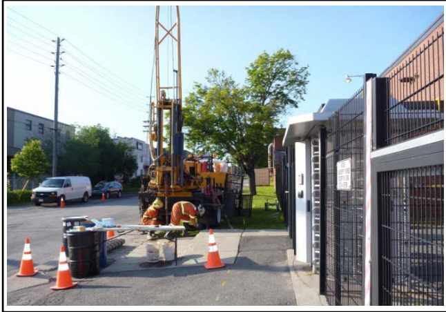
Photo 5 - Drill Rig Setup at MW3
