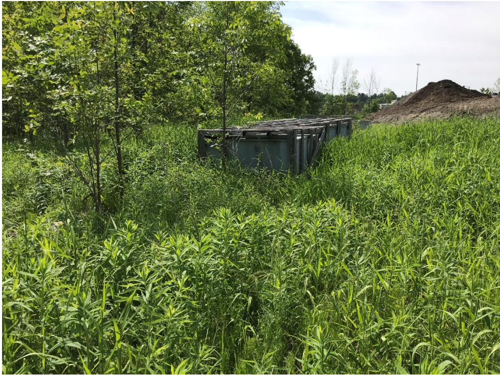
Photo 8 – View of two discarded roof supply fans on east side of Property; view is facing southeast.
