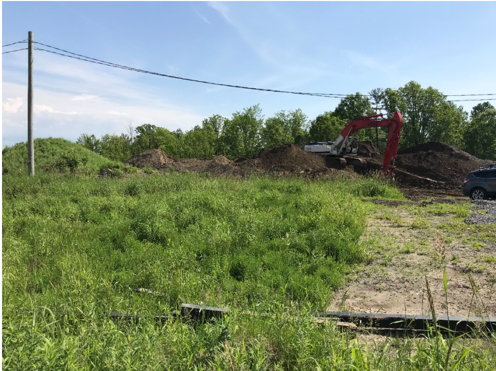
Photo 2 – View of two stockpiled fill materials (topsoil and sand); view is facing east.
