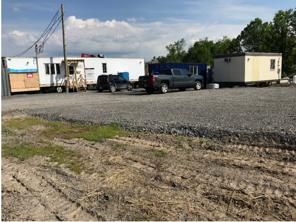
Photo 1 – View of the site trailers, C cans and gravel pad; view is facing northeast.
