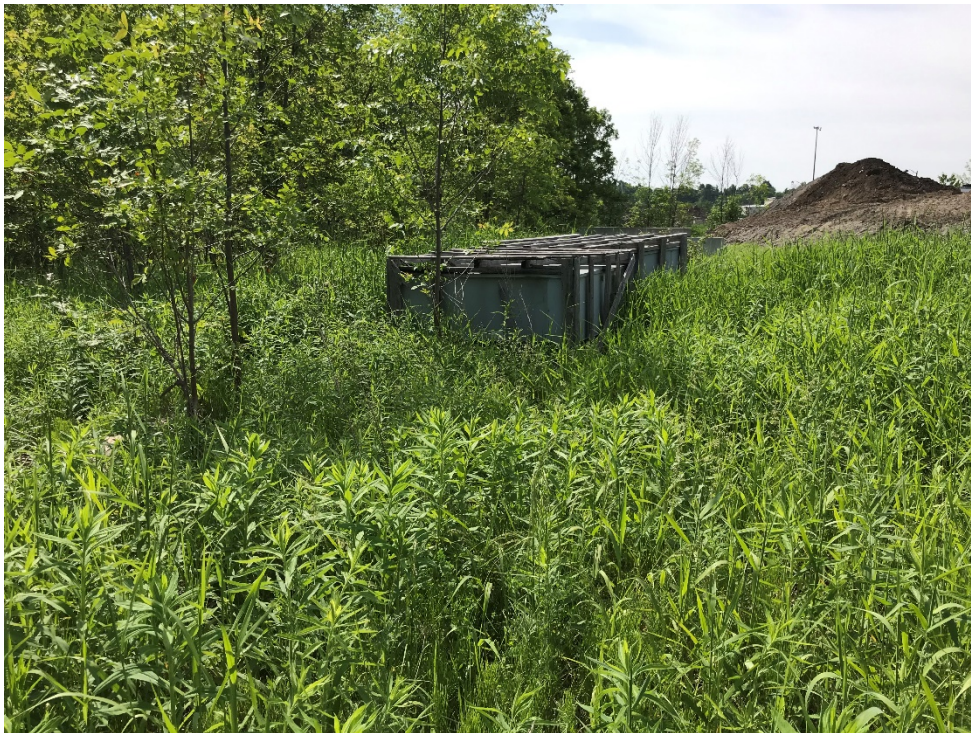
Photo 8 – View of two discarded roof supply fans on east side of Property; view is facing southeast.
