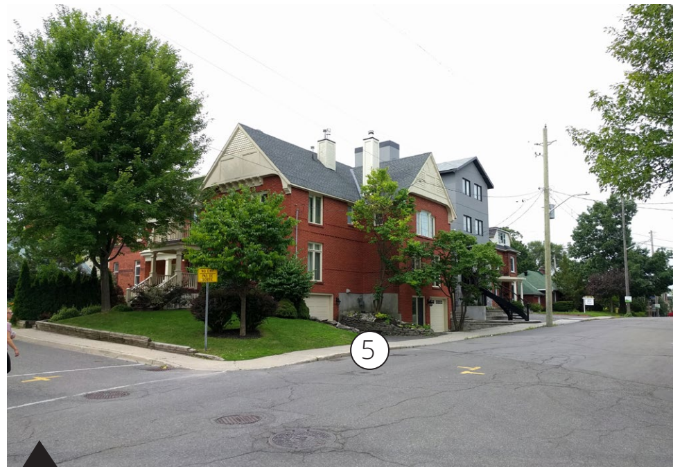
D AYLMER AVENUE CORNER GALT STREET / VIEW TOWARDS SOUTHWEST
