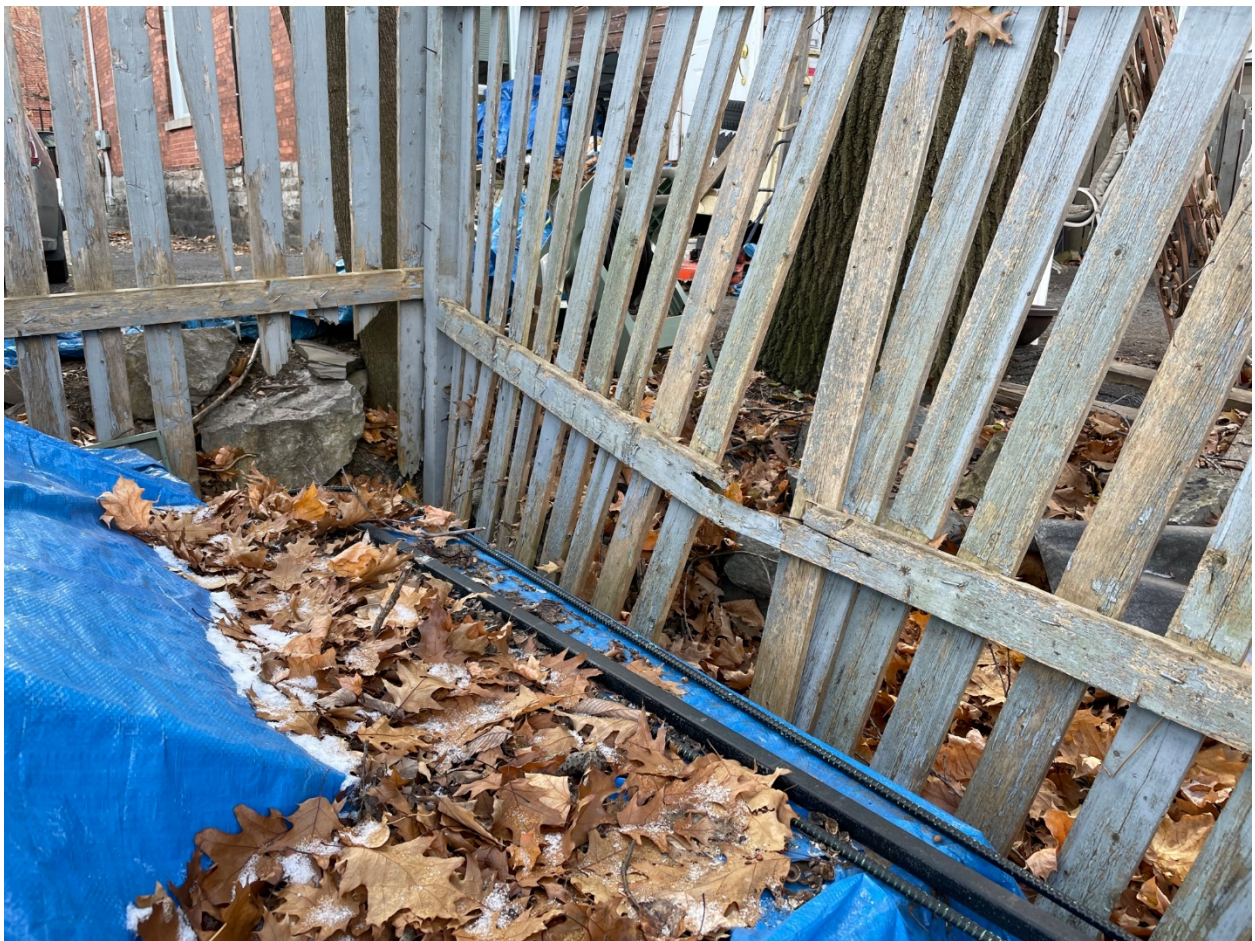
Figure 3: Photo taken from the Bank side demonstrating the 80 cm grade change right beside the tree
