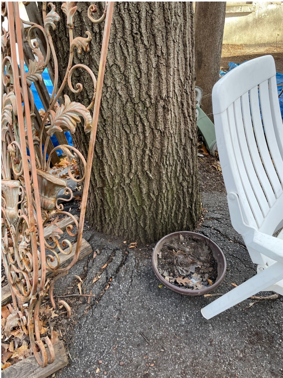
Figure 2: Photo showing how the asphalt is girdling the base of the tree
