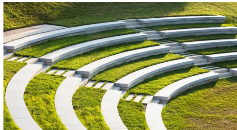
INTEGRATED CONCRETE SEATING WITH STEPS
