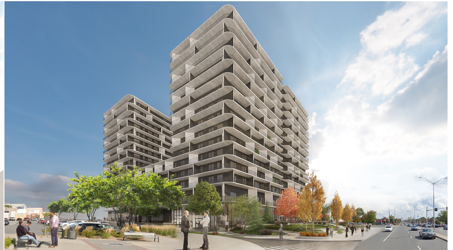
3. Street view of northern access roadway and Clyde Avenue
