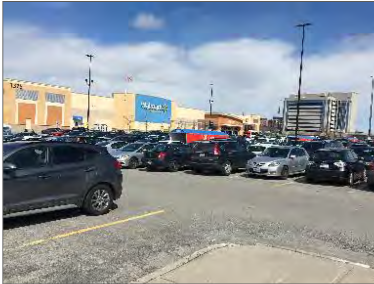
Photo 9 – Properties located east of the Phase One Property.
