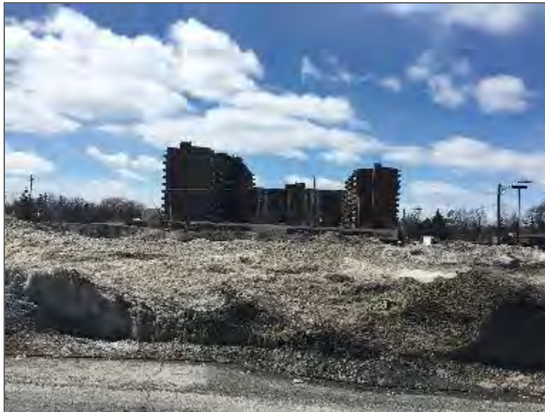
Photo 2 – View from the east boundary of the Phase One Property, looking west.
