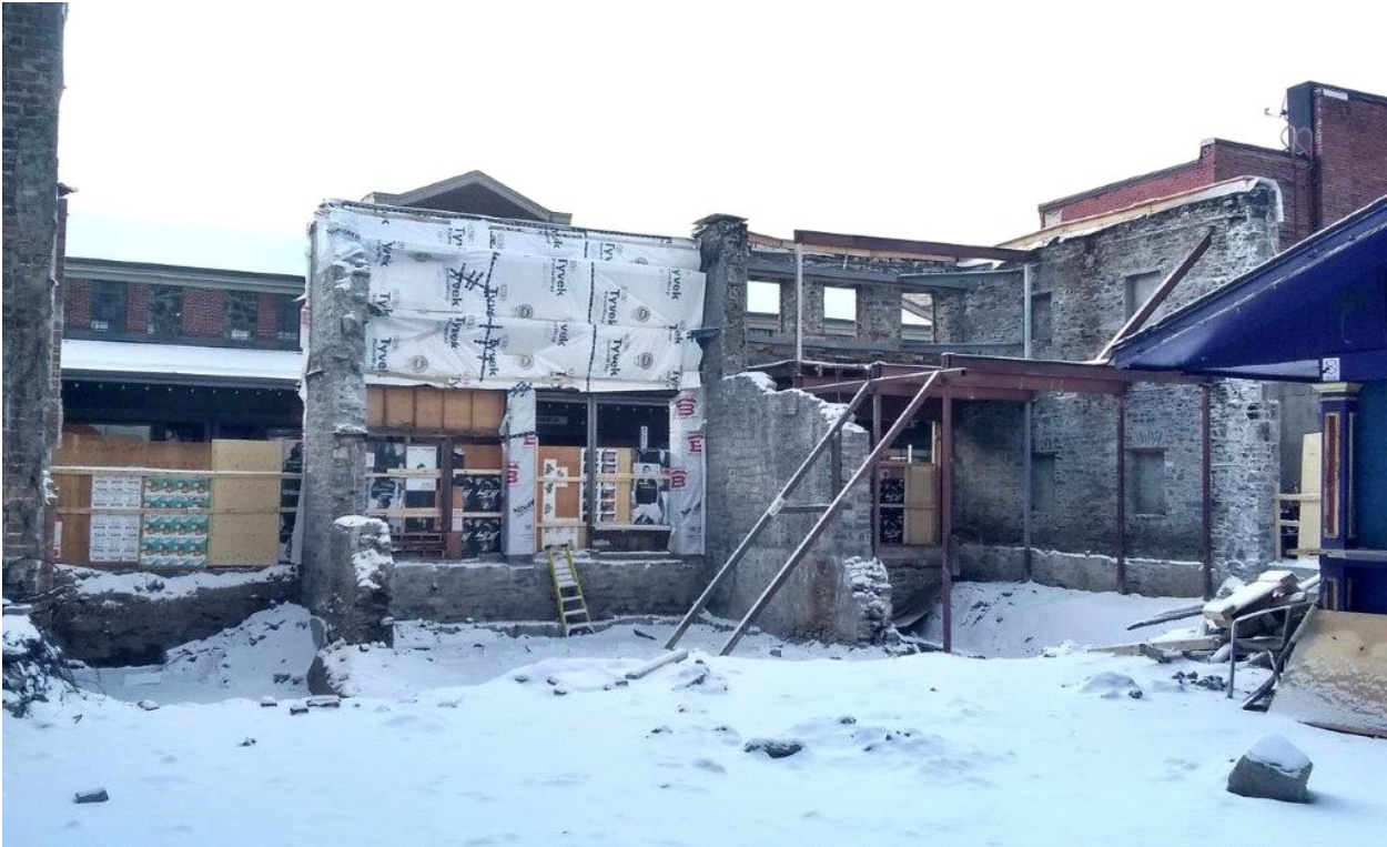
Figure 2. Photo taken facing William Street. Note that none of the former structure on the plan view above remains, except the façade.
