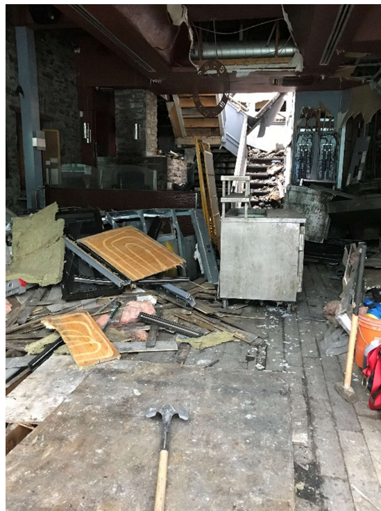
Photograph 2: View of the interior of 35-37 William Street, facing east.
