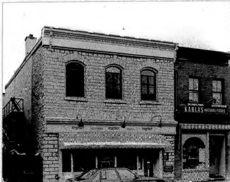
Attach building photos here: 1 - 6 x 6
