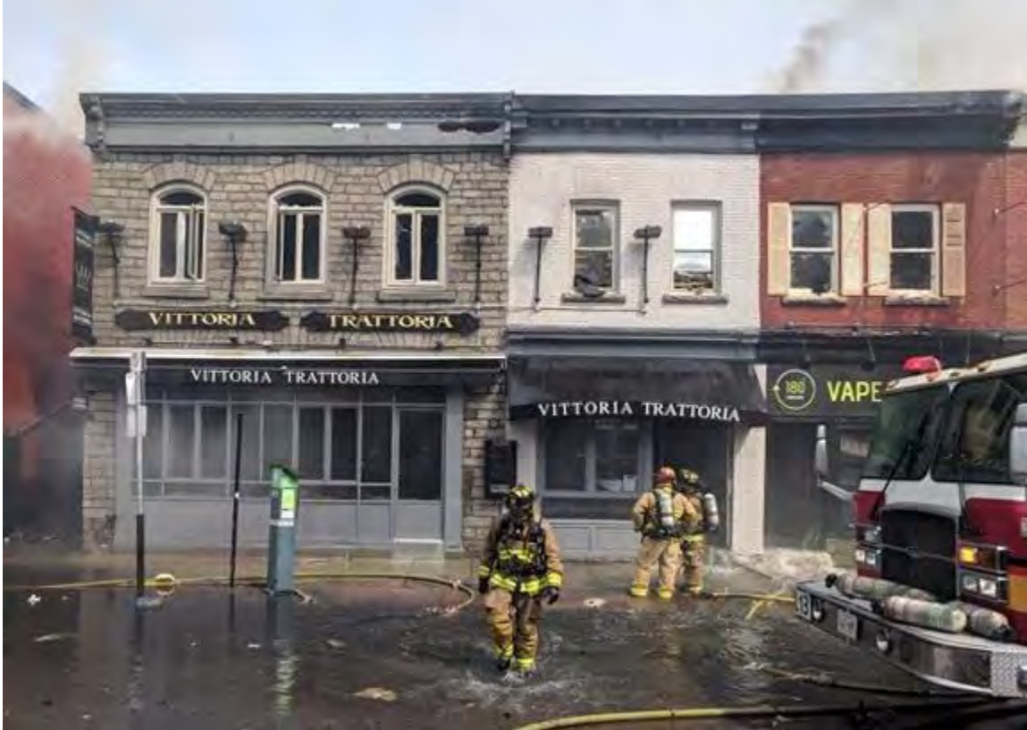
Figure 8: Fire at 35 William Street, April 12, 2019. Scott Stilborn/ Ottawa Fire Service
