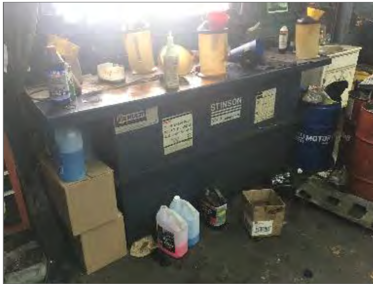
Photo 13 – A 1,008-L new oil AST located along the north wall of the tenant space occupied by Gifford's Automotive.
