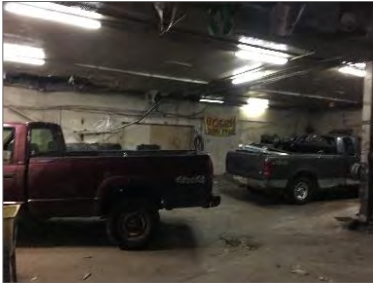
Photo 7 – Former automotive repair/servicing operation (i.e., Auto Re-Bex) within the north portion of Site Building A.
