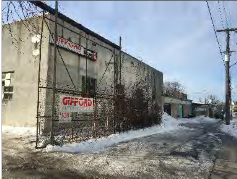
Photo 3 – Site Building A (east elevation).
