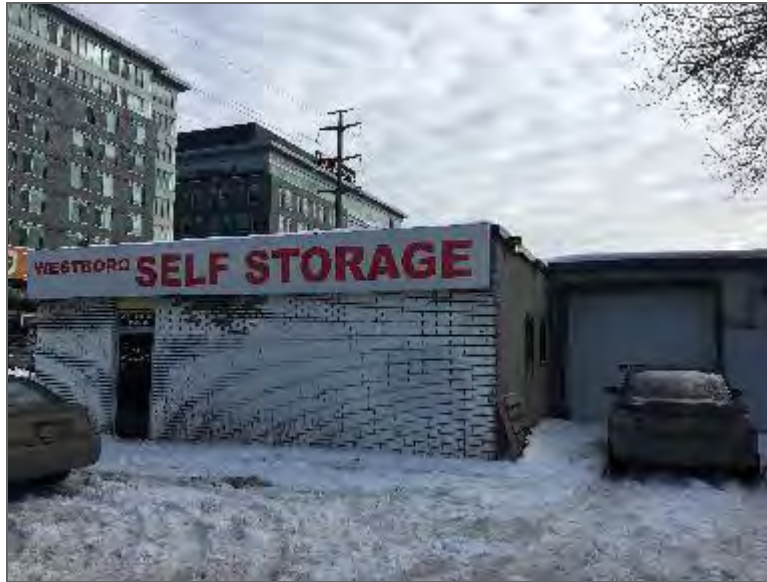
Photo 1 – Site Building A (north elevation).
