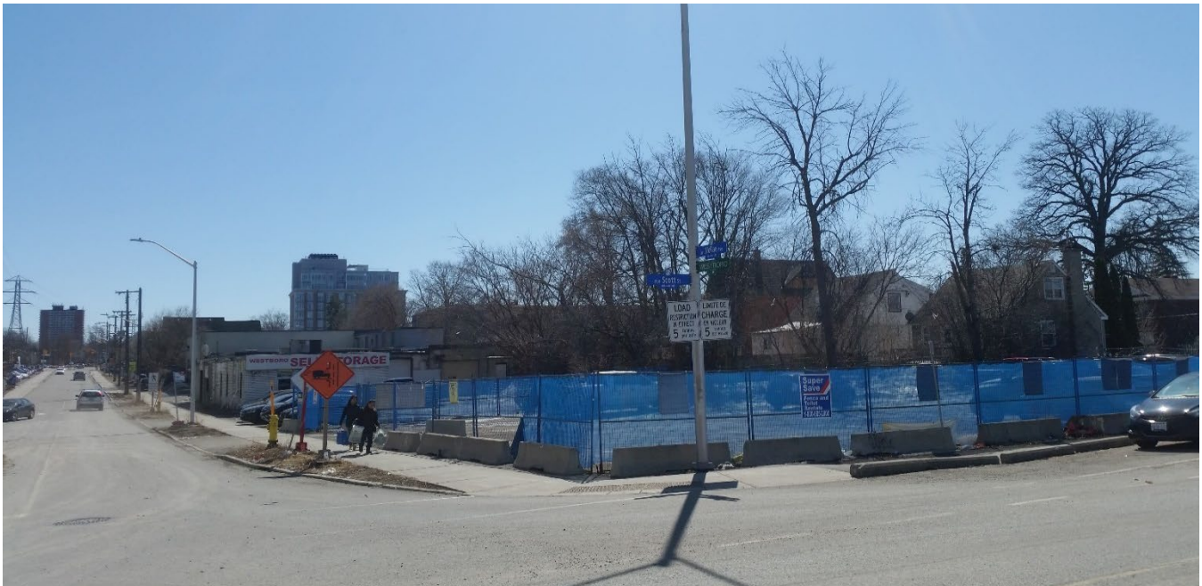
Figure 1. The Site Looking Southwest from Scott Street
