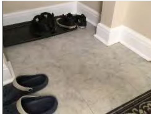
Non-asbestos peel and stick vinyl floor tiles present in the front entrance at 311 Tweedsmuir Avenue. Asbestos-containing vinyl sheet flooring is present underneath, as the base layer.
