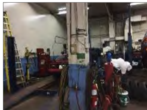
Asbestos-containing drywall joint compound present as the column finish in Garage 2 at 320 McRae Avenue.
