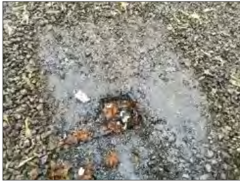
Non-asbestos built up roofing at 320 McRae Avenue.
