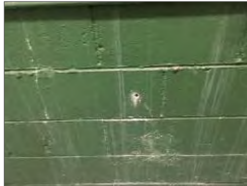
No vermiculite was present in the block walls at 320 McRae Avenue.
