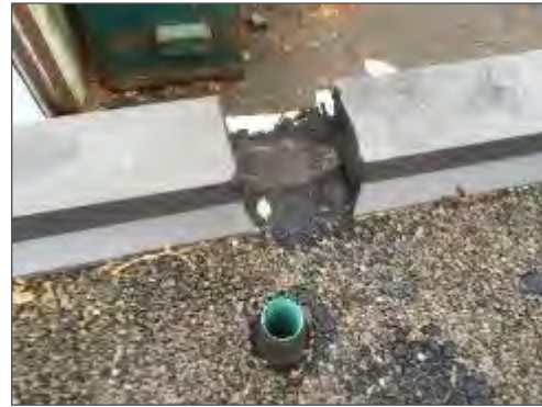
Non-asbestos tar on the roof at 320 McRae Avenue.
