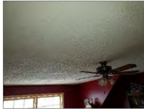
Non-asbestos ceiling stipple present throughout the second floor at 315 Tweedsmuir Avenue.
