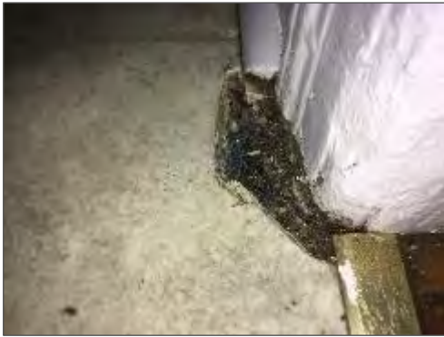
Asbestos-containing vinyl sheet flooring present in the multi-layered flooring at 311 Tweedsmuir Avenue.
