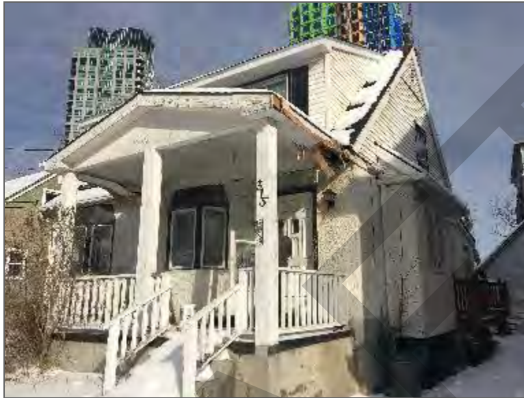
Photo 5 – View of Site Building C from Tweedsmuir Avenue.
