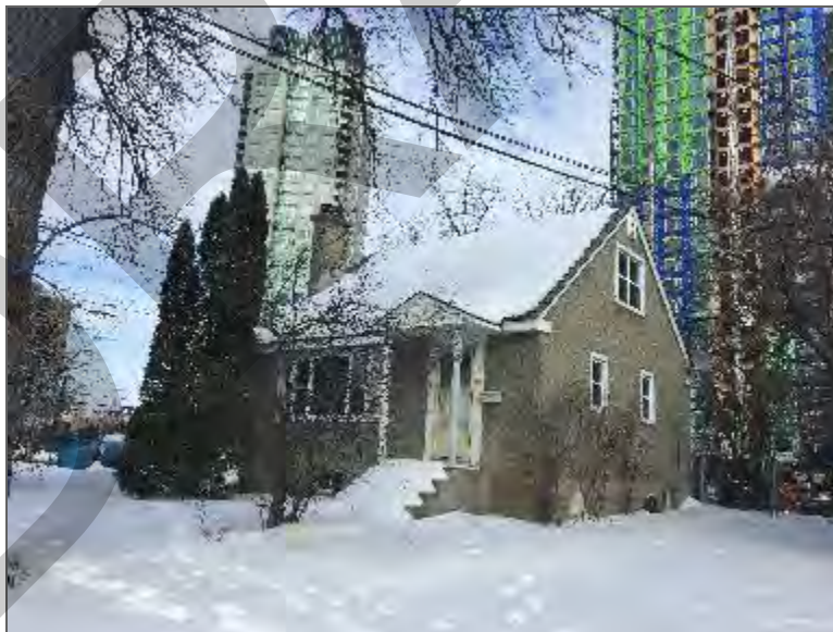
Photo 4 – View of Site Building B from Tweedsmuir Avenue.
