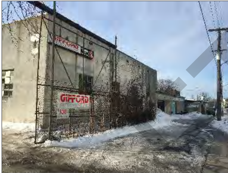
Photo 3 – Site Building A (east elevation).
