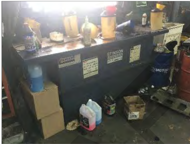
Photo 13 – A 1,008-L new oil AST located along the north wall of the tenant space occupied by Gifford's Automotive.
