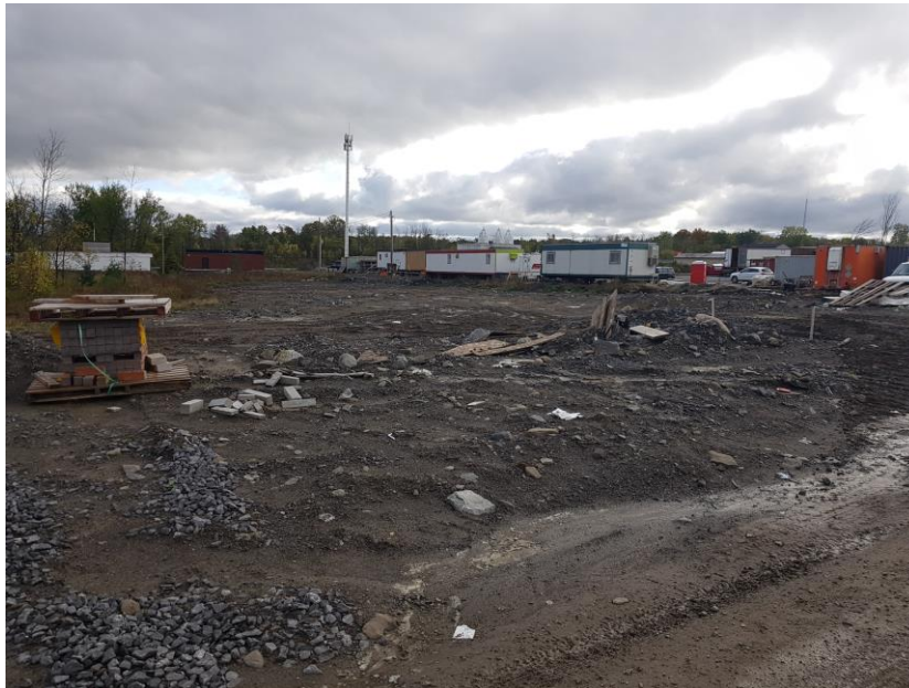
Photo 2 – Construction Staging east of the Site, east of Cedar Creek Drive
