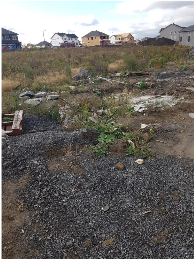
Photo 5 – Construction debris located on Site
