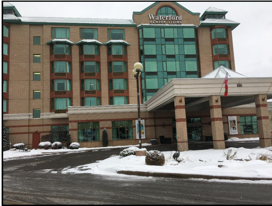
Photograph 1: Southern (front) view of the subject building, looking north.
