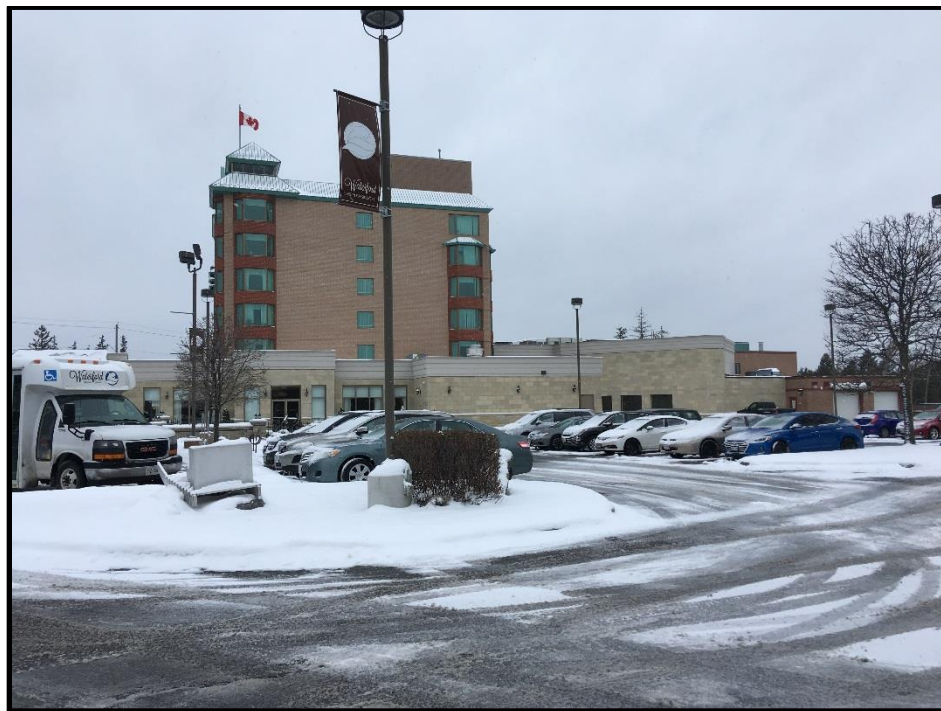
Photograph 4: Central east view of the Phase I Property, looking west.
