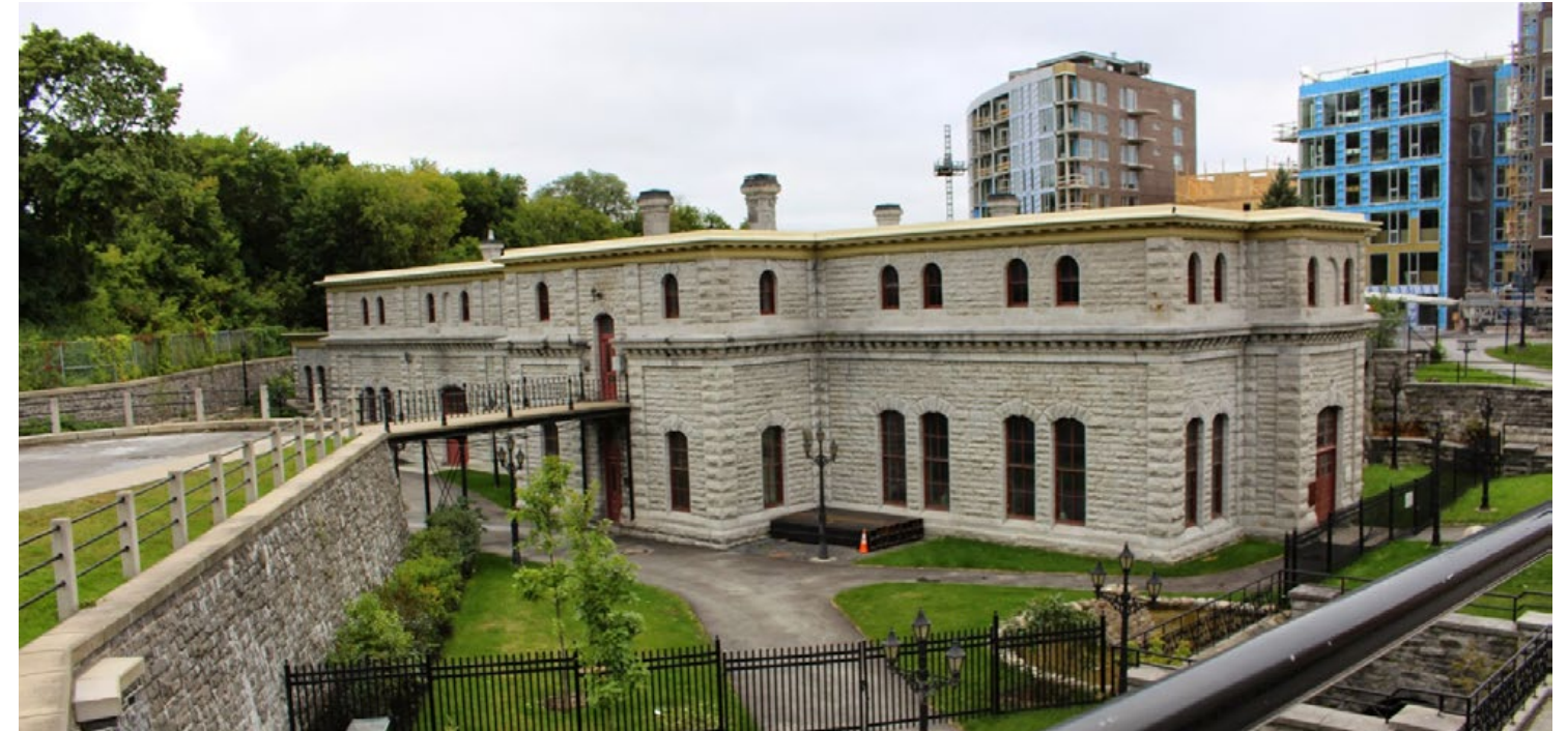
The Fleet Street Pumping Station
