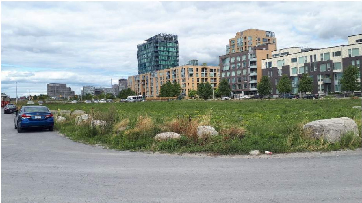
Photograph 2: View of the subject site looking north from the corner of Lett Street and Lloyd Street.
