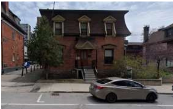
Figure 10: 494 Albert Street, main elevation. Source: Google streetview, May 2019.
