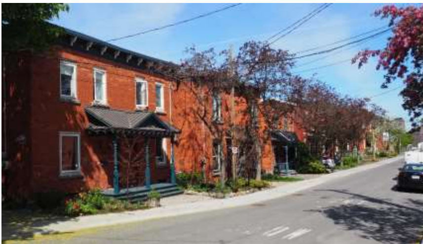
Figure 12: Lorne Avenue (west side), in the Lorne Avenue HCD. Source: Contentworks, 2020.
