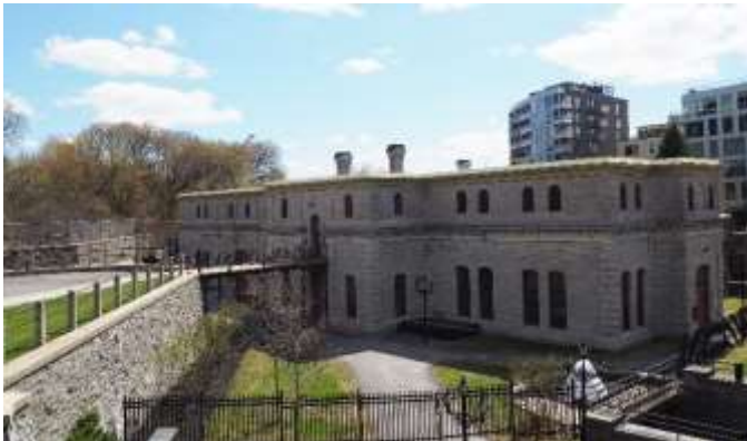
Figure 7: Ottawa Water Works Building. The proposed development will sit on the bluff behind the building. Source: Contentworks, 2020.
