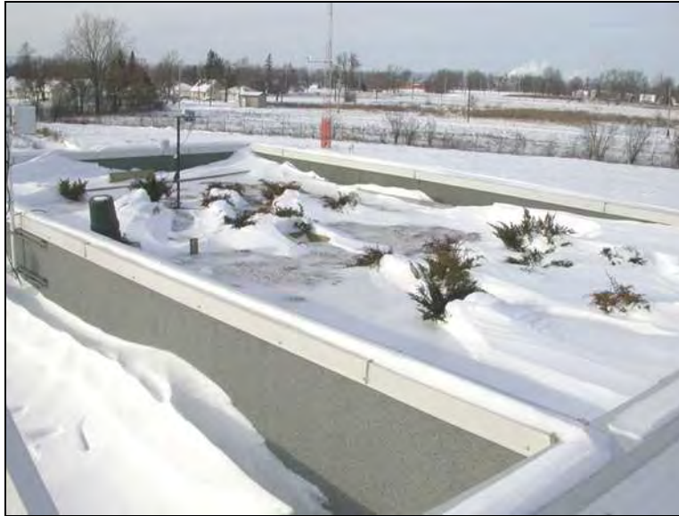
Figure 4.2.2 A green roof during winter
