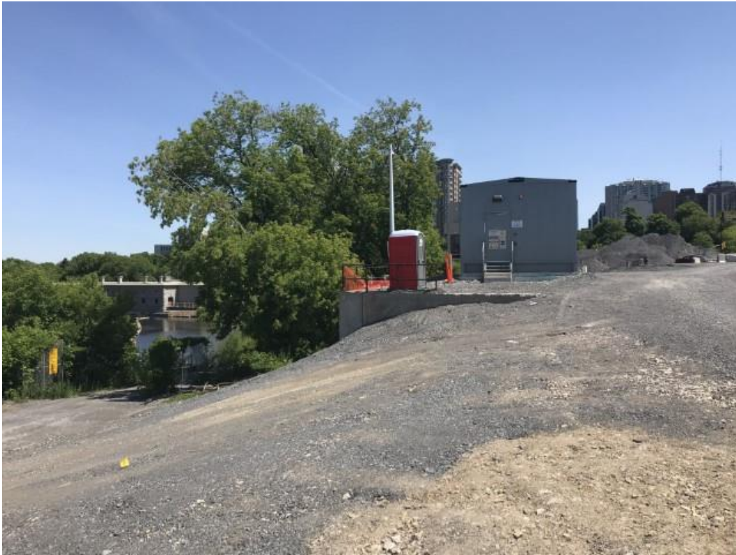
Photo 9: Grade change between Site (right) and aqueduct (left)
