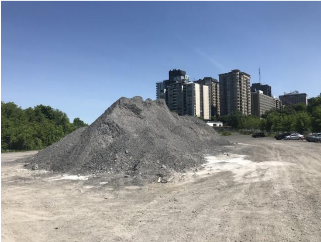
Photo 1: Site looking northeast
