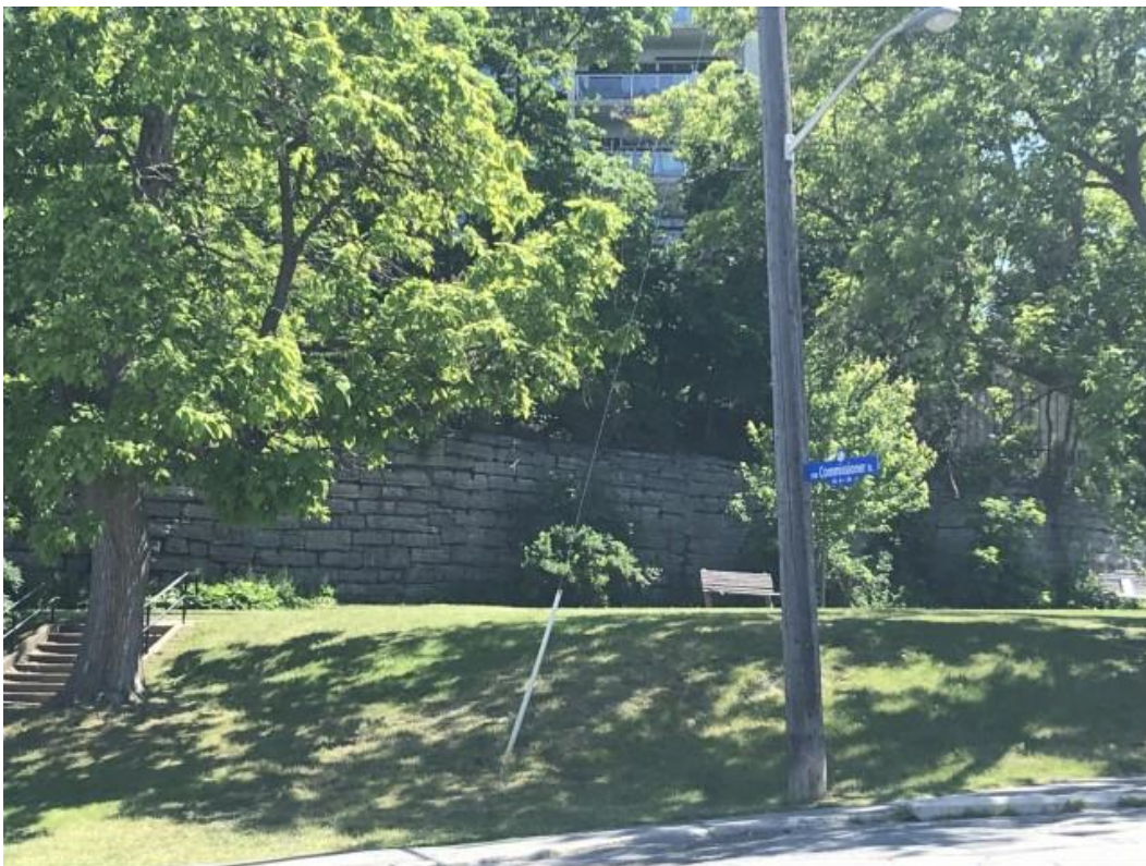
Photo 2: Stone retaining wall at Area 2 north of Site
