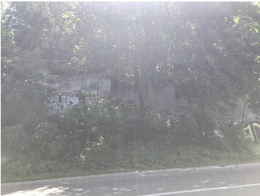
Photo 12: Retaining wall in Area 3 east of Slater St.
