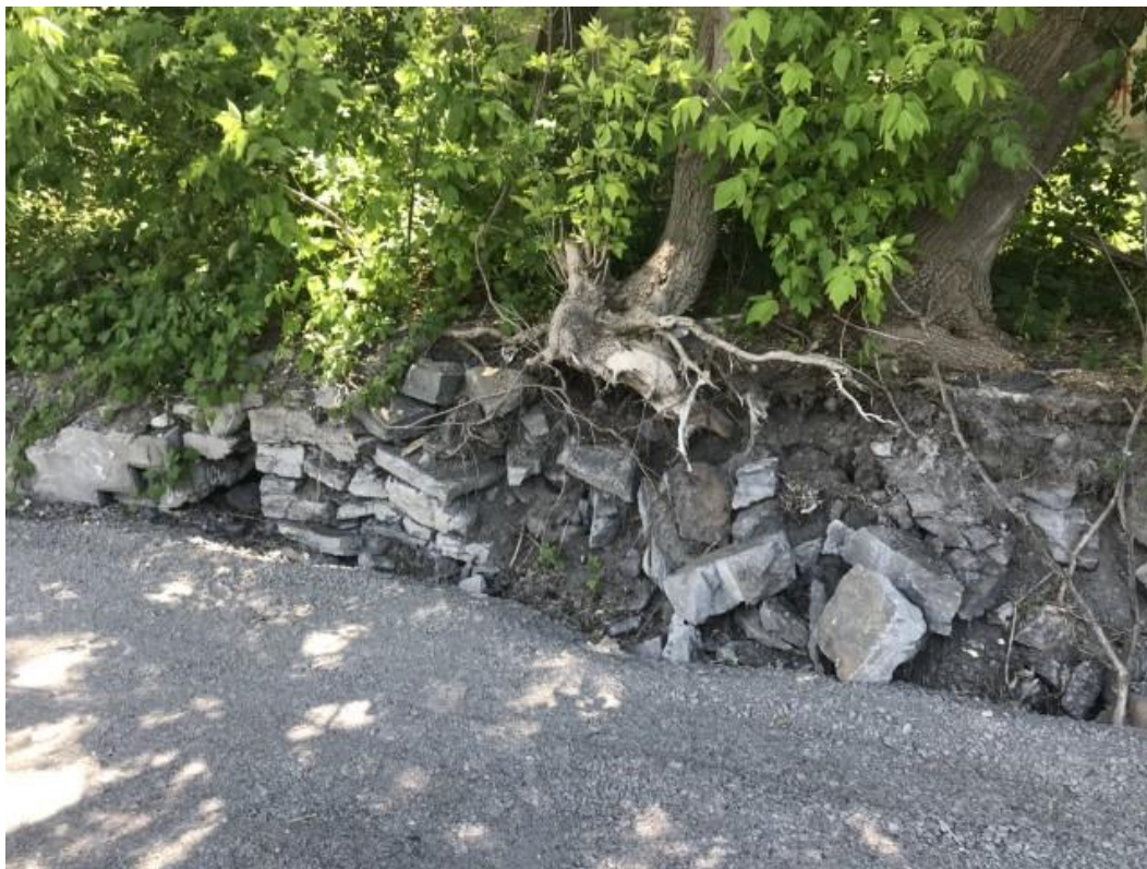
Photo 8: Retaining wall in Area 1 along aqueduct, west of Site
