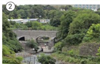
Pooly's Bridge & Pump Station
