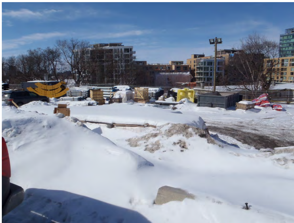
Photograph 8: Overview of laydown/storage area west of the water treatment system buildings.
