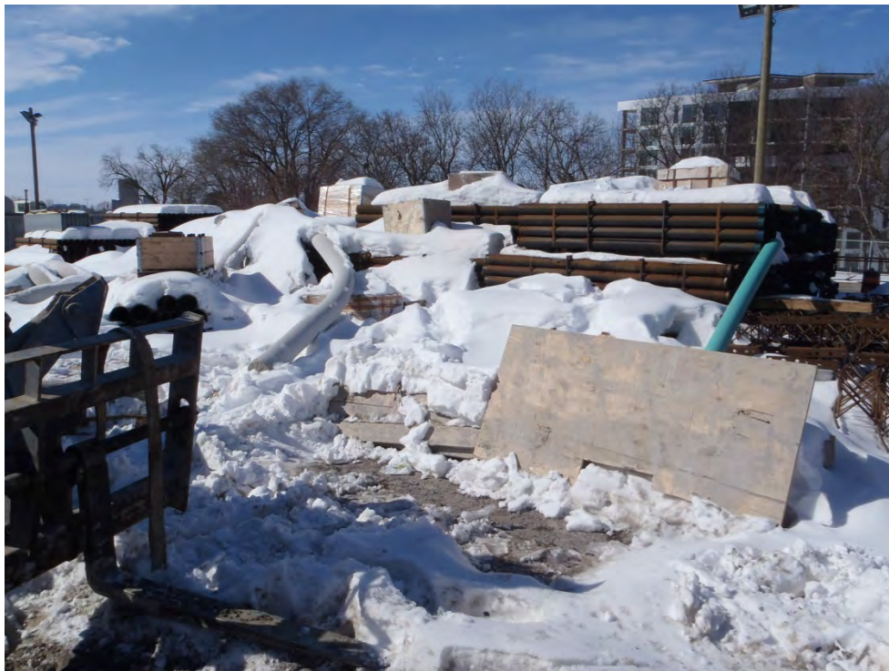
Photograph 10: Materials/equipment storage located along the north boundary of the Site.
