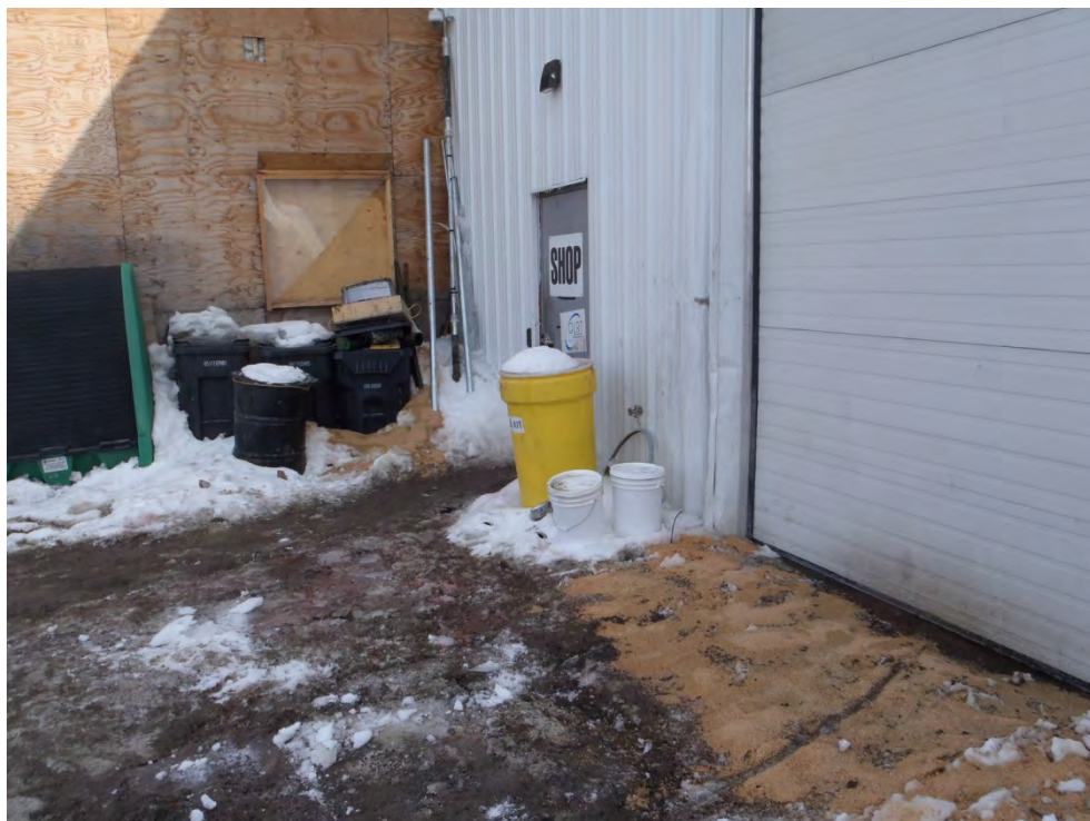
Photograph 22: North entrance of the shop/garage with noted absorbent material on the ground and around a tote. This is a noted area where spills have occurred.
