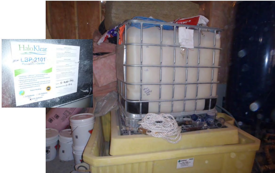
Photograph 4: HaloKlear LBP-2101 Flocculant/Clarifier stored in 1,243 L tote with secondary containment.
