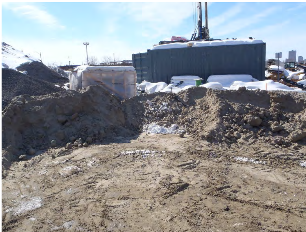
Photograph 12: Looking southwest towards subcontractor sea containers and fill pile (left).
