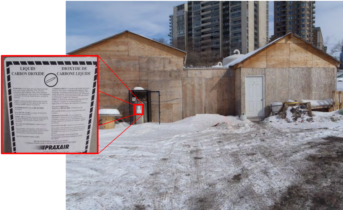
Photograph 3: Water treatment system building located in the north corner of the Site. Tank of liquid carbon dioxide located in a cage outside the water treatment system building.
