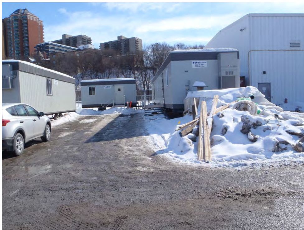
Photograph 16: Site trailers located to the northeast of the shop/warehouse/garage building.
