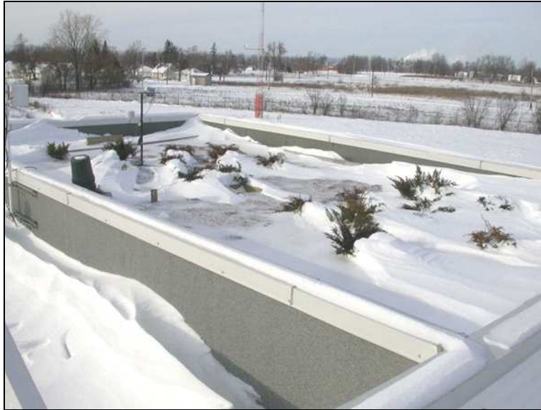
Figure 4.2.2 A green roof during winter
