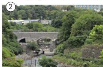
Pooly's Bridge & Pump Station
