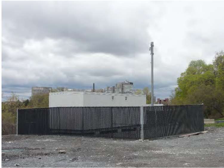
Photo 3 – View of the parcel of land occupied by temporary pre-fabricated building for telecommunication infrastructure on the northwest portion of the Site, looking northwest.
