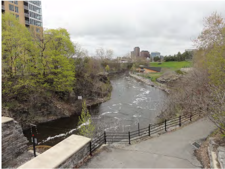
Photo 11 – View of a portion of the aqueduct located west of the Site.
