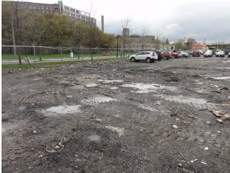
Photo 5 – Approximate location of former garage building with chemical storage tanks at the Site, looking southeast (no evidence of stain or spills observed).
