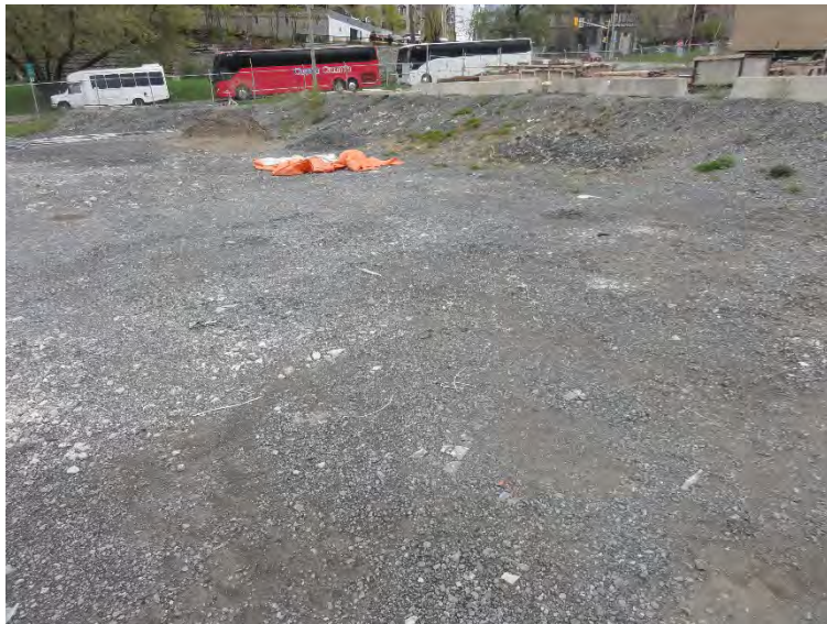
Photo 4 – Approximate location of former water treatment system on the northern portion of the Site, looking northeast.
