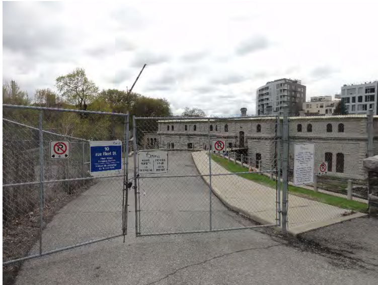
Photo 9 – View of the Fleet Street Pumping Station located west of the Site at a lower elevation, looking southeast.
